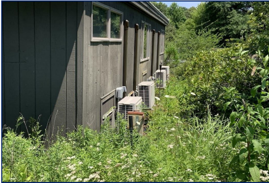
Adkins Arboretum, HVAC Installation $40,000
