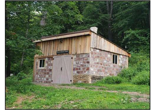
Evergreen Heritage Center, Appalachian Coal Camp Project $25,000
